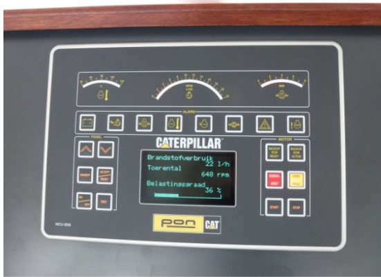
Fuel meter in wheelhouse
