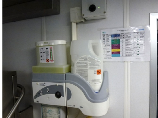
Automatic dosing system for cleaning chemicals
